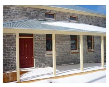
The first phase of the Kiandra Courthouse restoration included re-establishing the verandah and the removal of the paint to expose the original brickwork (photo by Jennifer Hewitson).
